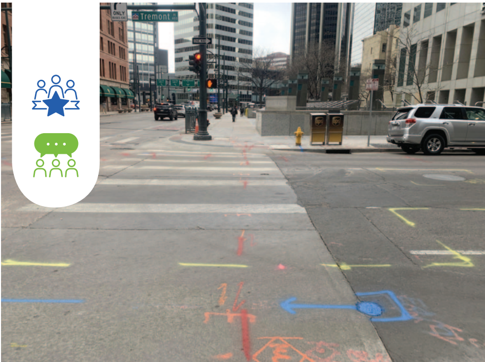
Lines and symbols painted on the ground near Tremont Street in downtown Denver, Colo. communicate important safety information used by construction workers to avoid damaging underground water, natural gas, electric and communication lines.
