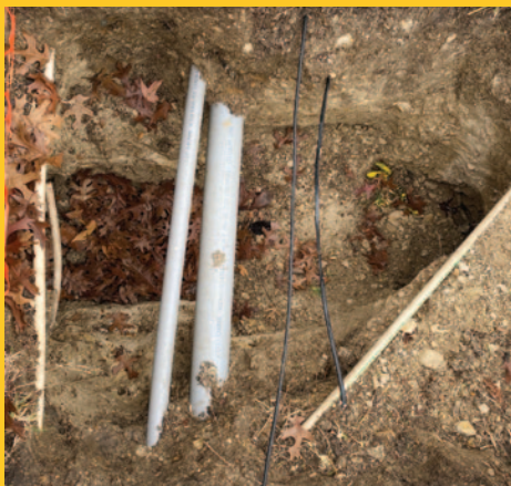
Quality Level A (QL-A) data collected through Subsurface Utility Engineering (SUE) surveys involves physically exposing underground facilities and utility lines to collect precise horizontal and vertical positional data.
